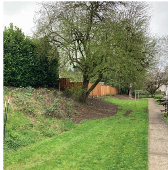
Southern Retaining Walls
